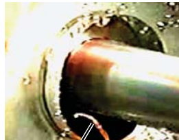
Water Being Pumped into the Bearing Cavity
